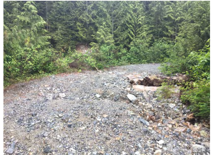
Approach from Right Bank when facing downstream
